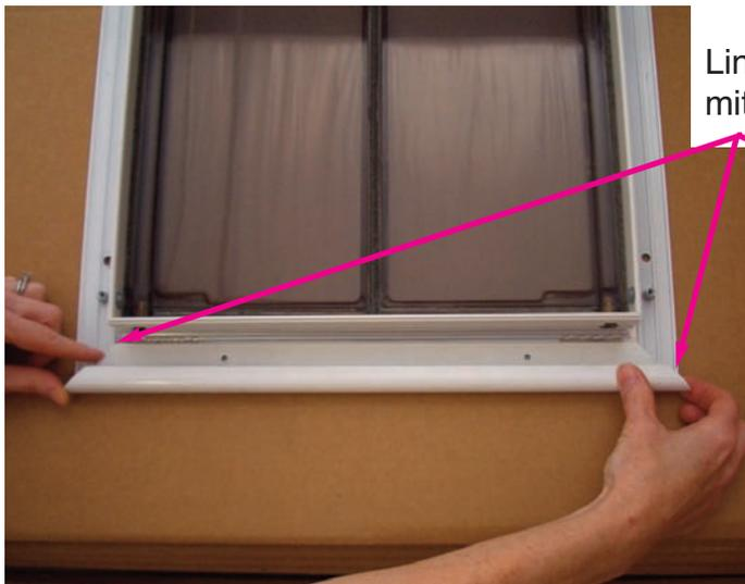
Line up bottom slide track piece with mitered corner joints.
