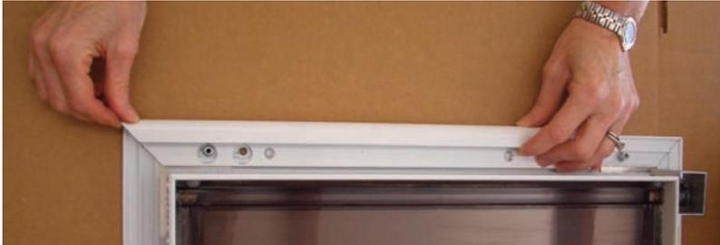
Align first side piece with mitered joint and then mark screw holes with fine pointed marker, as you did with the bottom frame. Again, check that the screw hole marks are in the center of the frame track. Then repeat for final side piece.
