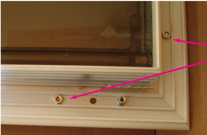
Close-up view of back of pet door frame after holes have been drilled and slide in track frame pieces screwed in place and LocTite put on back of bolts.
